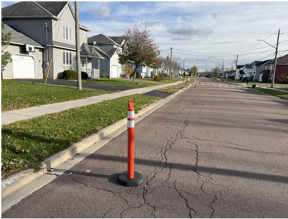
Photo 1: Beginning of Litter Site
